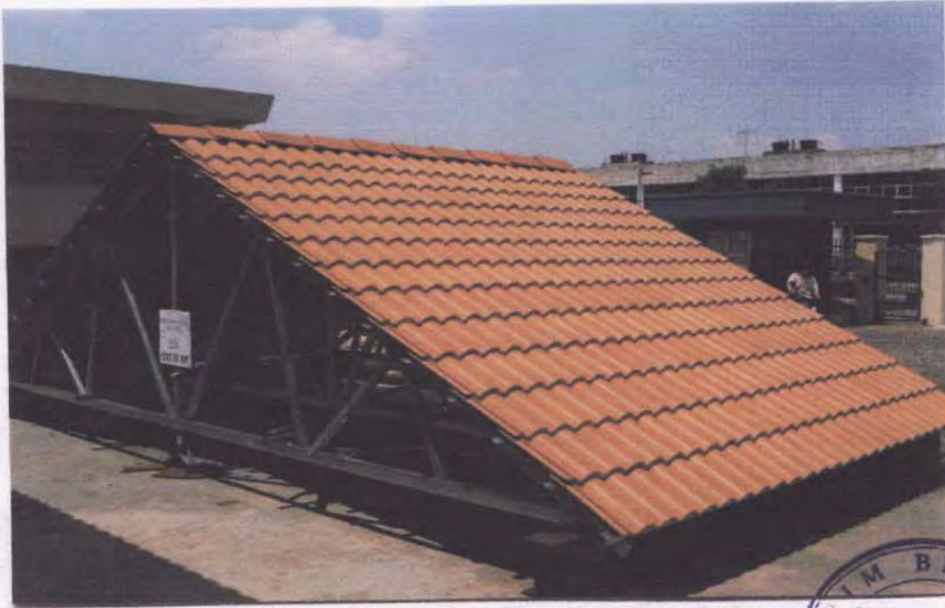
Deflections were recorded after a layer of roofing tiles were fully assembled on the steel roof truss.
