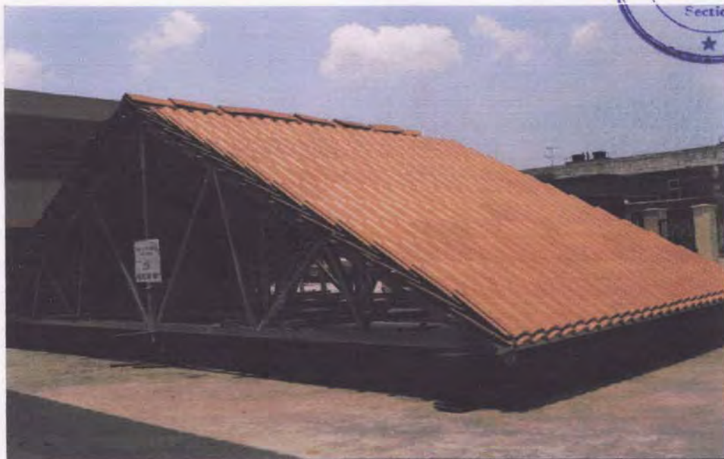
Deflections were recorded after two layers of roofing tiles were fully assembled on the steel roof truss.
