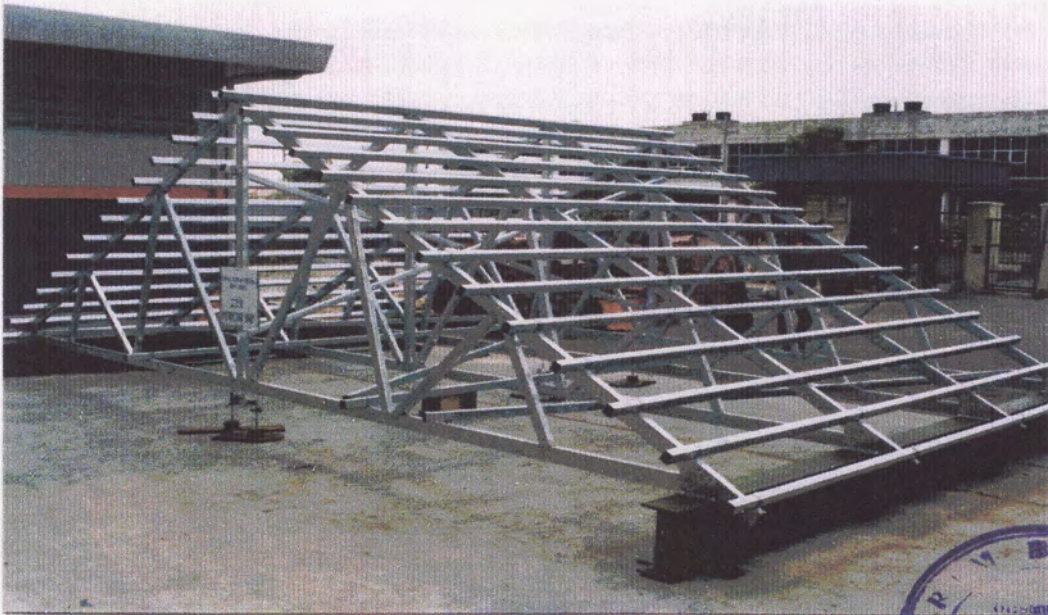
Steel roof truss assembly.
