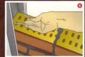
Special wire brick ties comes with each metal door frame. These ties are for bonding the brickwork.
