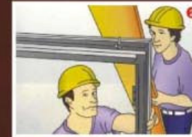
To prop up metal door frame, use two planks with nails at the ends. Ensure the correct direction of your door hinge then stand up the door frame. The nails on the plank should hook the edge of the frame.
