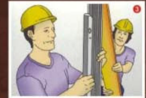
To check whether the frame is properly plumbed, use the spirit level.
